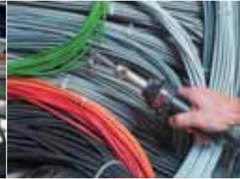
Fitting a solder shrink connection with HOT JET S and push-fit sieve reflector.
